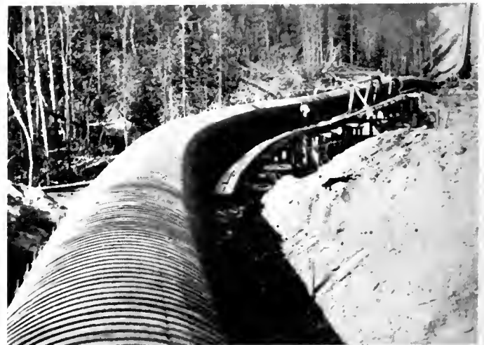
Fig. 5—66" Wood Stave Pipe Syphon, Kamloops Power Plant.
